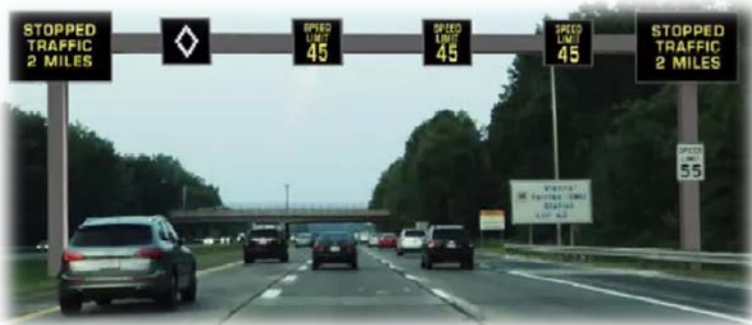
Highway and tolling systems
