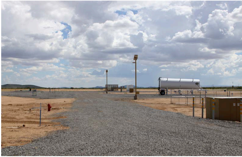
WASTEWATER TREATMENT PLANT
