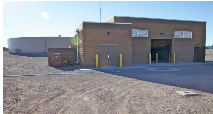
1.3M GAL WATER STORAGE & BOOSTER STATION
