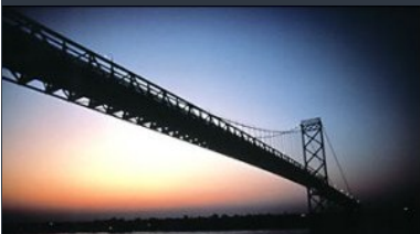
Ambassador Bridge, Detroit, MI
