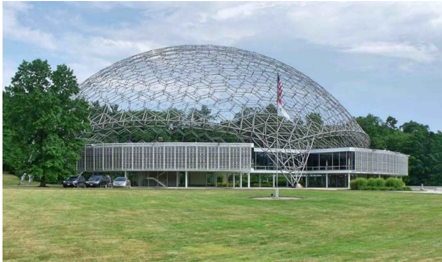
Figure 2 Geodesic dome, over ASM Headquarters
