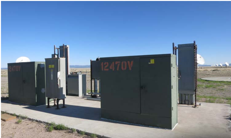
Updated medium-voltage electrical services, foundation anchors, grounding, and fiber optics
