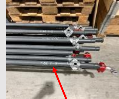
4. Arranging pipes in numbered order
