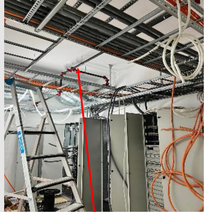
Installed Sprinkler system with Re-work
